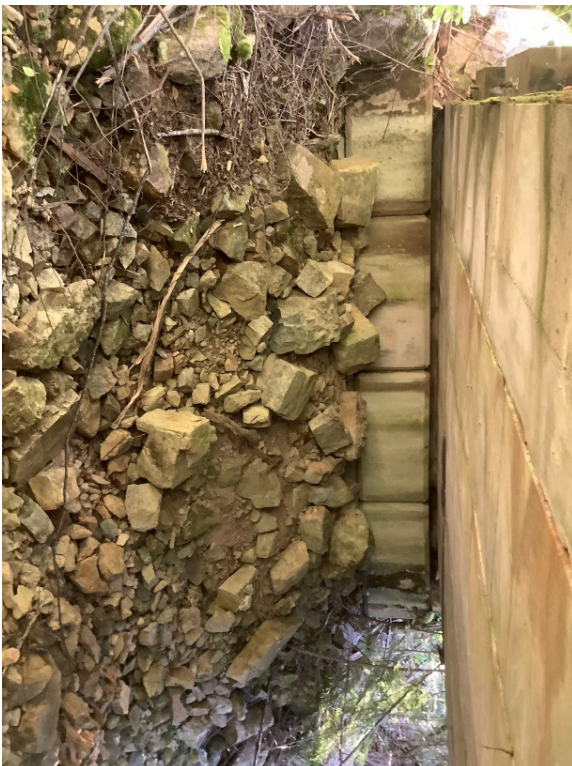
Left Bank Abutment when facing downstream
